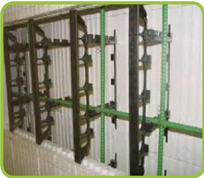
Example of webs with steel fixing.
