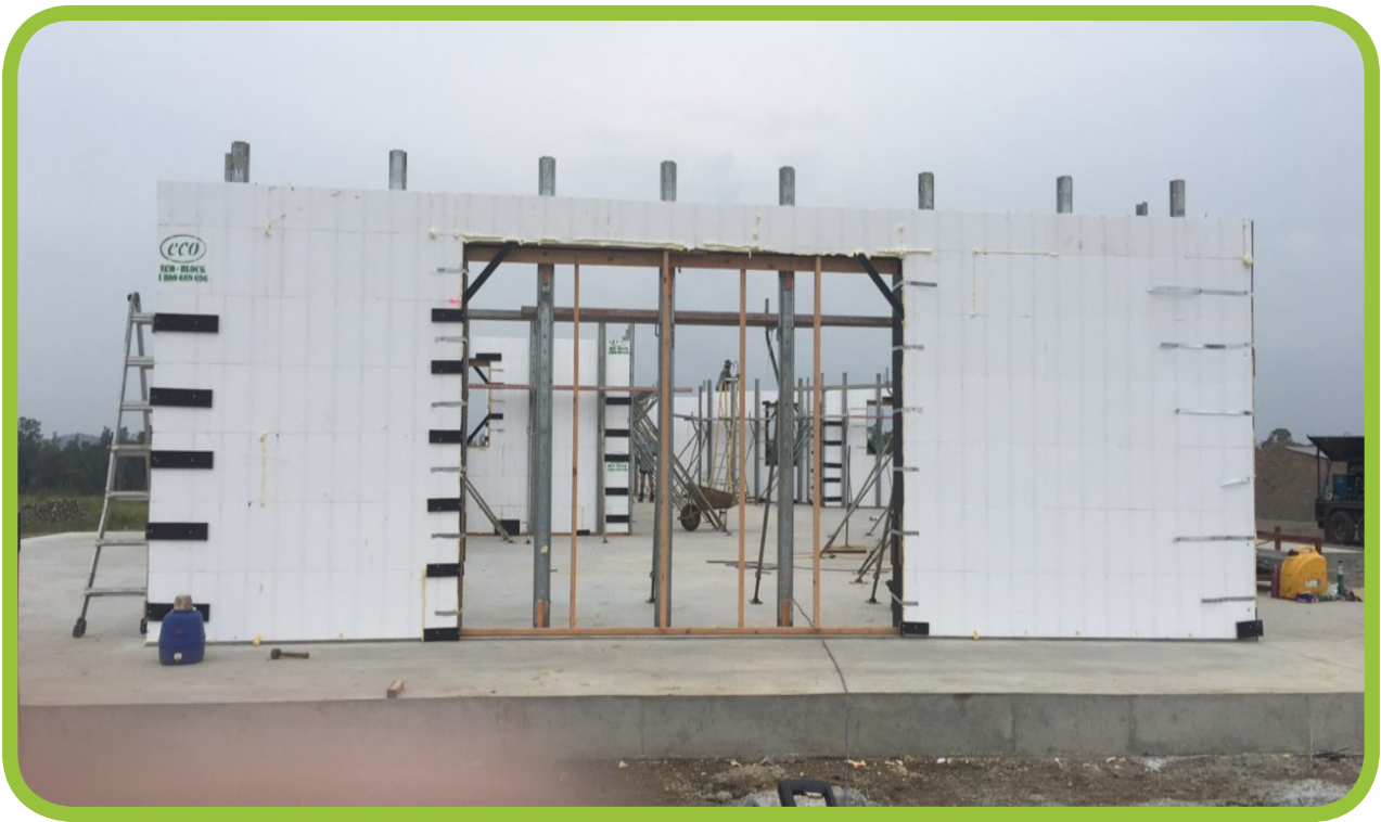
Formwork doors and windows secure
