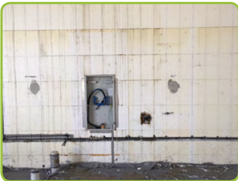
Electrical box fitted in walls before the concrete pour.
