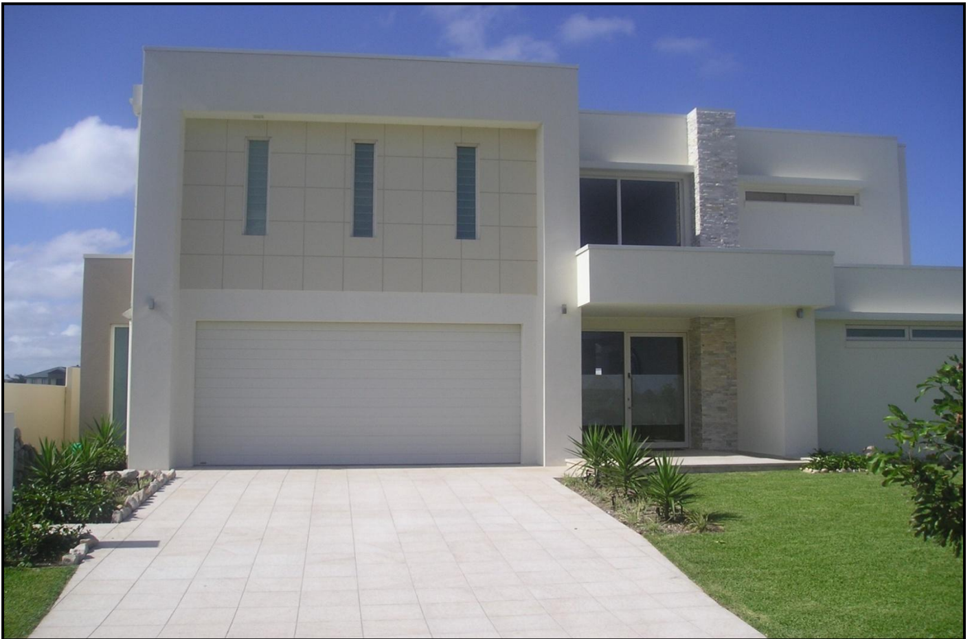
Completed ICF Home
